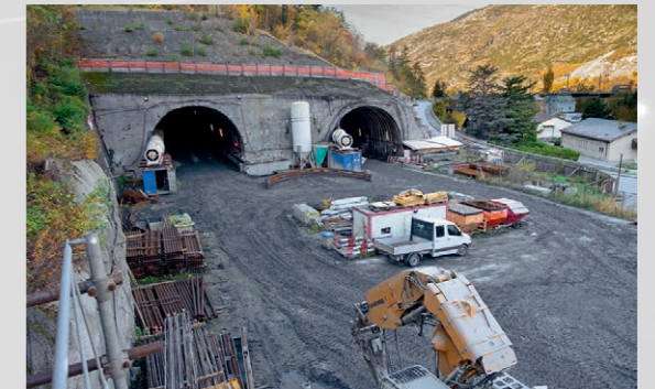
Tunnelportal Ost Tunnel Riedberg.
