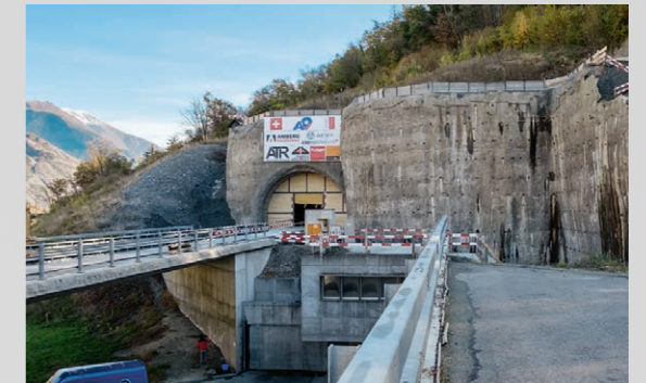
Tunnelportal West Tunnel Riedberg.
